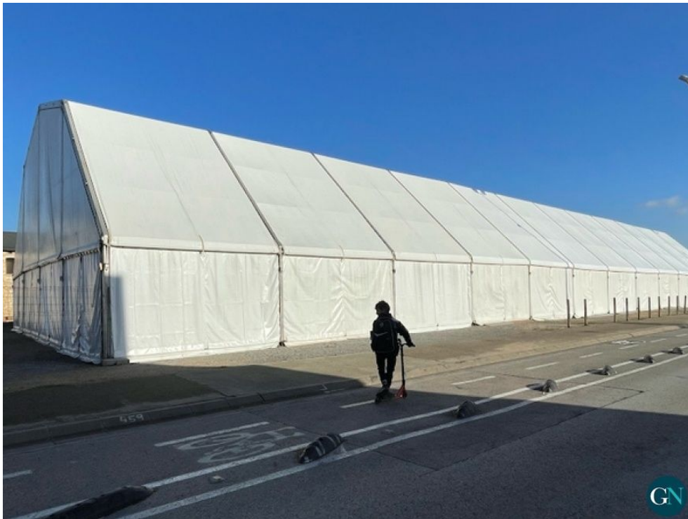
Envelat de 1.200 metres quadrats
